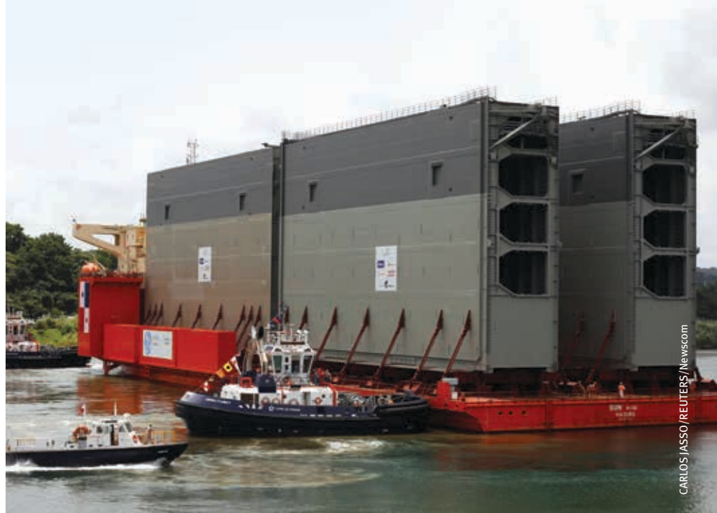
The first four new gates for the Panama Canal's third set of locks are seen on top of a cargo ship during their arrival to Colon in Colon City on August 20, 2013. The third set of locks has a total of 16 rolling gates, eight for each new lock complex.
