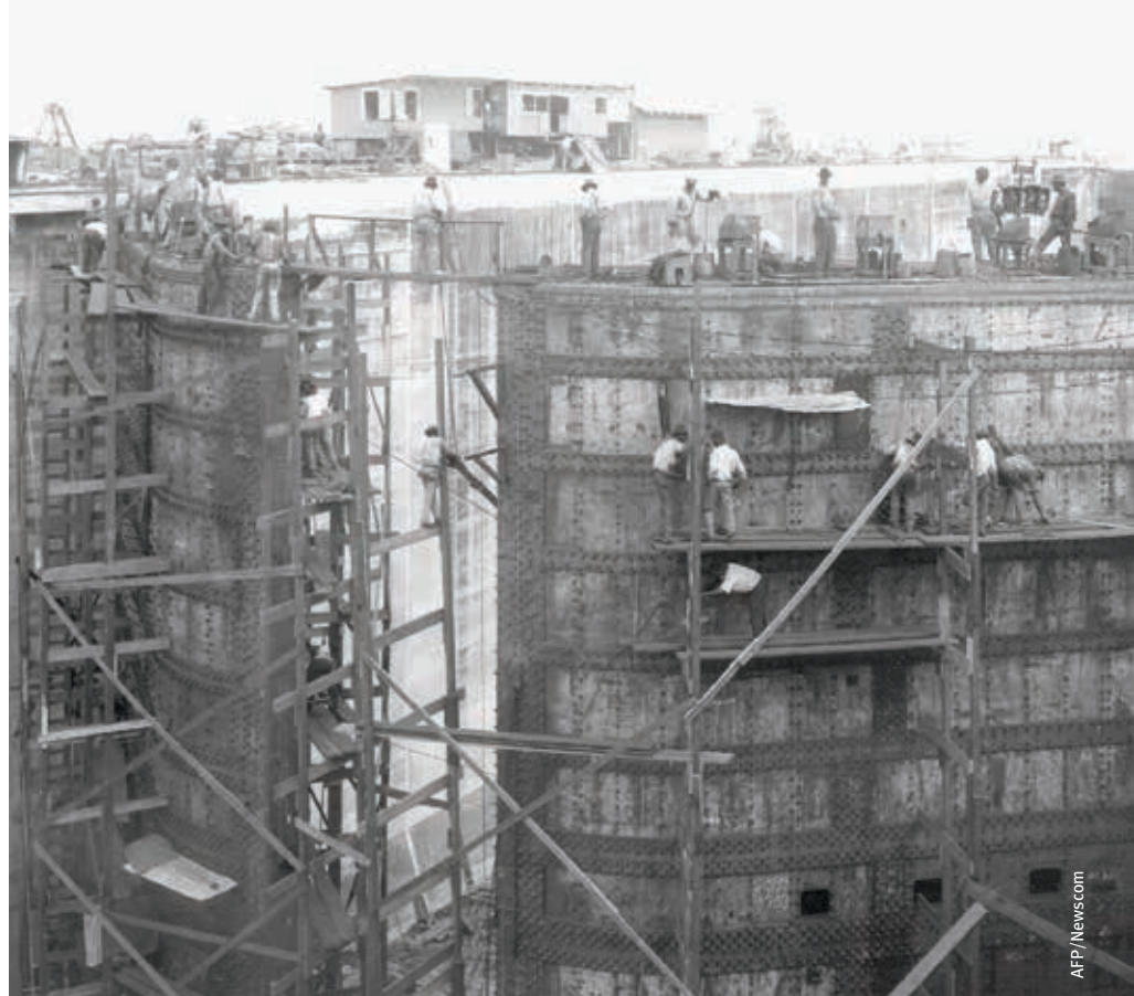
This undated file photo shows workers building one of the gates at the Gatun Locks on the Panama Canal. The canal has three locks: Miraflores and Pedro Miguel on the Pacific side and Gatun on the Atlantic.
