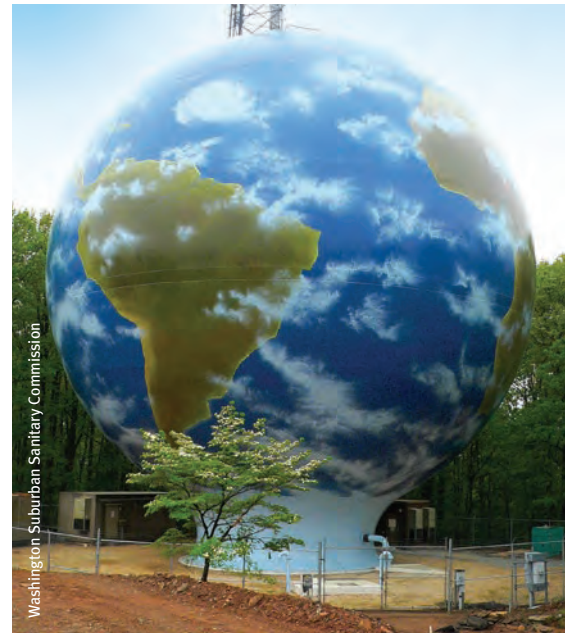
Water in a storage tank at the Washington Suburban Sanitary Commission, which provides water to more than 1.8 million residents in Prince George’s and Montgomery counties in Maryland.
